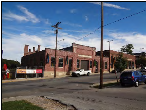
Fig. 3: south (front) elevation of the Agricultural & Industrial Museum (AIM)
