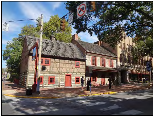
Fig. 9: south (front) elevations of the Golden Plough Tavern (left, at corner) and General Gates House (right) and 1920s-era commercial building at right
