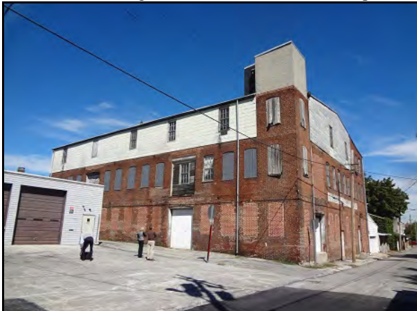
Fig. 13: south and west elevations of Clarke Warehouse
