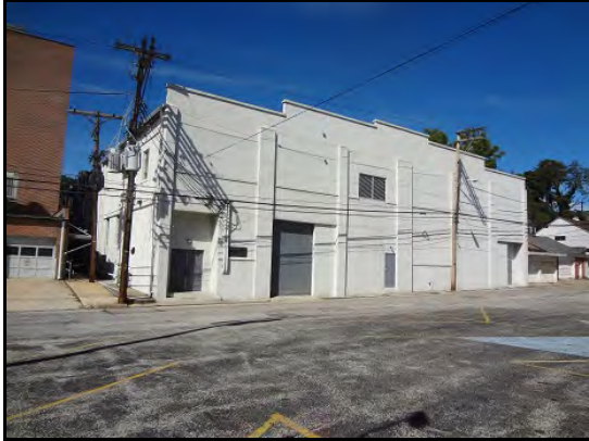
Fig. 19: south (rear) elevation of the Historical Society Museum building. Several parking spaces are currently available at the rear of the Baker Building (the brick Building to the left in the photo)
