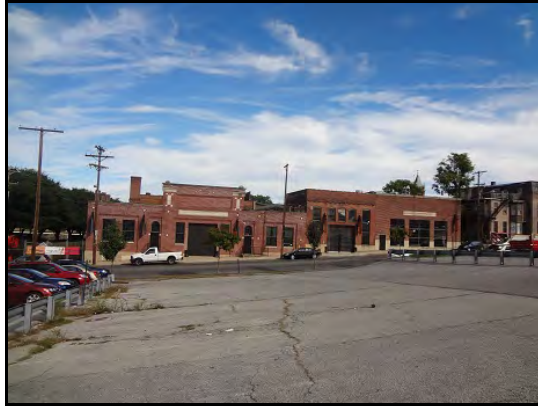
Fig. 20: long view of south (front) elevation of AIM taken from the high school parking lot; there are 10 spaces for AIM at the left side of the photo (behind the guard rail)
