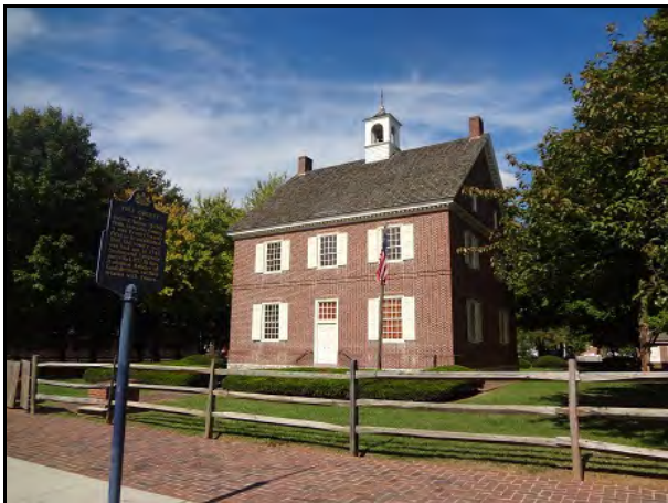
Fig. 11: south elevation of Colonial Court House directly west of N. Pershing Avenue in the Colonial Complex
