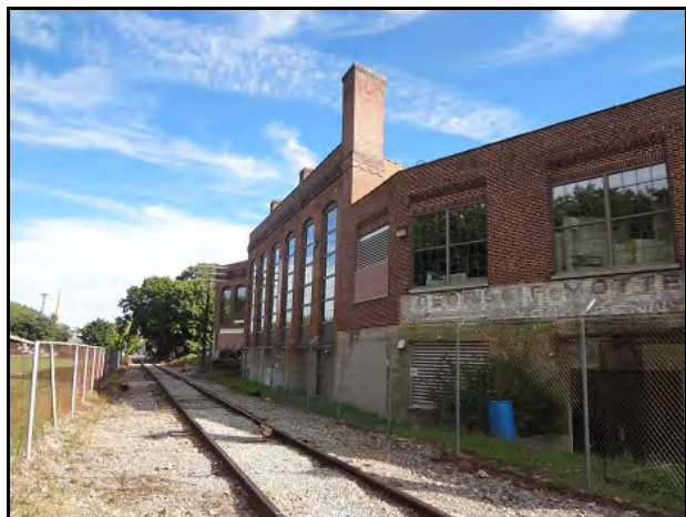
Fig. 18: view north along the railroad track at AIM looking toward the Colonial Complex – two blocks away.
