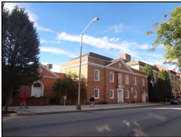
Fig. 1: north (front) elevation of the Historical Society Museum and Library/Archives Building ( all photos in this report by J. Bowie )
